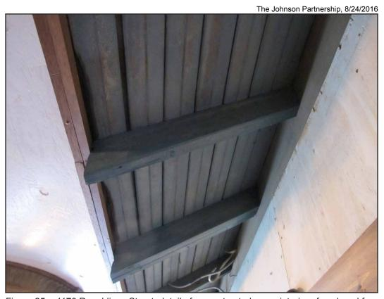
Figure 25 • 1170 Republican Street, detail of reconstructed eave, interior of enclosed former side yard
